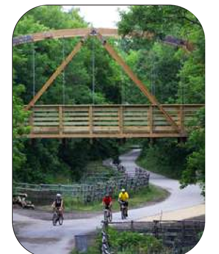
Expansion of the Lakeland Trails
