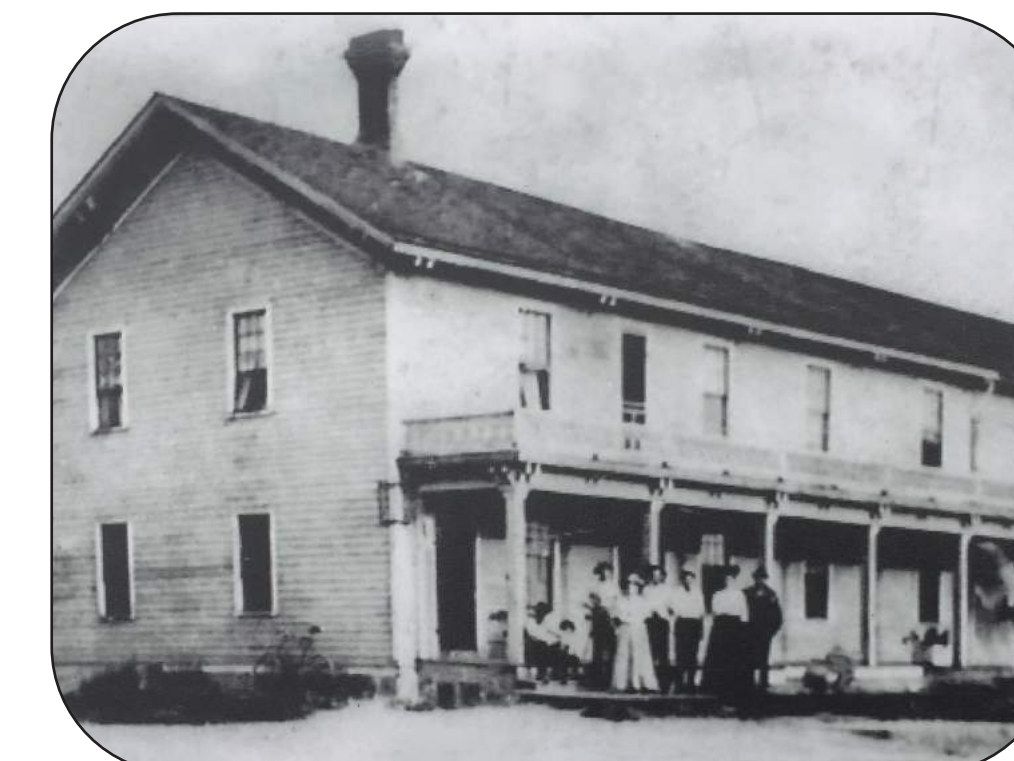
Hotel Inspired by the Winkelhaus Hotel (built in 1835, destroyed in 1968)
